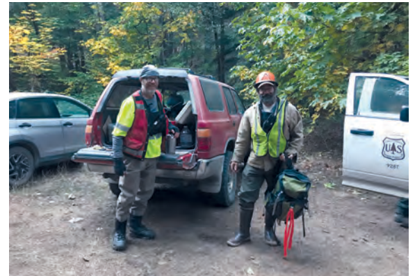
Charles Wickman and Rocco Fiori getting ready to start their day of directing the placement of logs for the Horse Helicopter Wood Loading Project. Photo taken on October 20, 2020.
