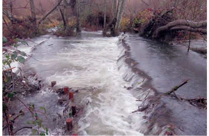
MKWC Fisheries led by Jimmy Peterson, installed a human made beaver dam to replace the one that was blown out in the winter of 2010/2011. This “beaver dam analogue” (human made beaver dam) connects Boise Creek to over a 1/2 acre of off-channel ponds that provide valuable summer and winter rearing habitat for salmonids.
