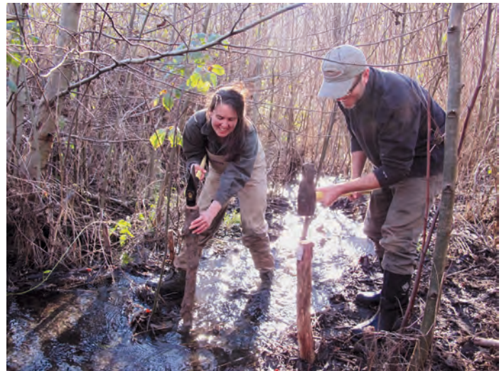
MKWC Fisheries personnel creating a beaver dam analogue on Camp Creek on January 6, 2011. We want to mimic beavers and the great work they do for our aquatic environment.
