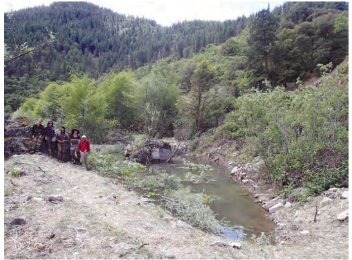
Tom Martin Creek on May 9, 2014 after adding brush bundles to the alcove connected to the creek. These bundles of brush provide cover for salmonids, increasing their chance of survival.
