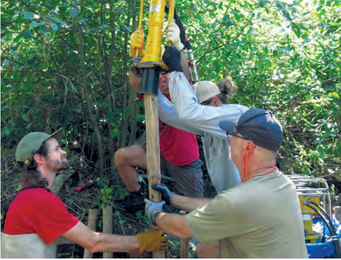
Installing a BDA at Boise Creek
