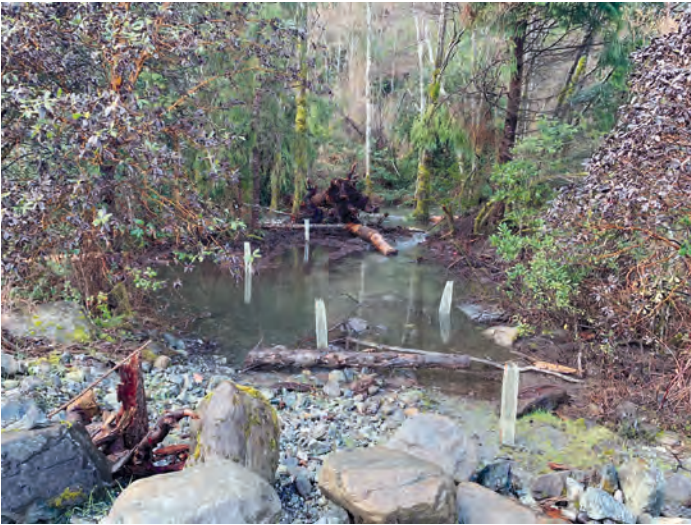
Aikens Creek wood structure on February 13, 2021. The wood structures installed in the summer of 2020 backed up high winter water for over a hundred feet pushing water up on the creek's floodplain and creating nice low velocity winter rearing habitat for salmonids.
