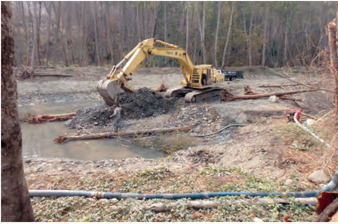
An off-channel pond being constructed on October 10, 2017.
