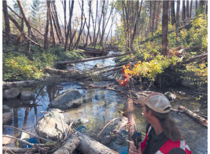
50 large logs with root wads were added to a 1/2 mile section of Horse Creek Valley in the fall of 2019. This photo taken on October 14, 2019 is looking downstream from the most upstream wood structure.
