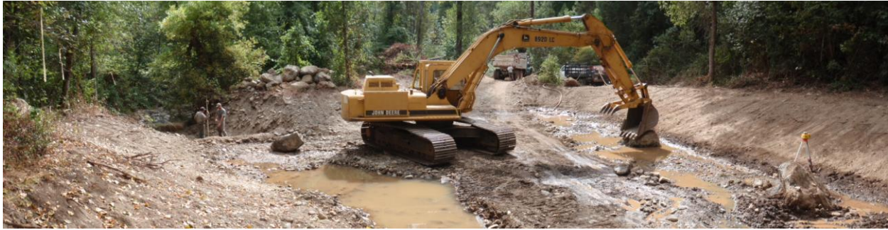
Figure 4. Panoramic view of off-channel pond at Stender property on Seiad Creek. The pond connects to Seiad Creek on the left and is fed by a perennial stream that goes subsurface 200 meters upslope of the pond. We anticipate beavers may inhabit this and other created ponds over time. Photo: Will Harling, MKWC.
