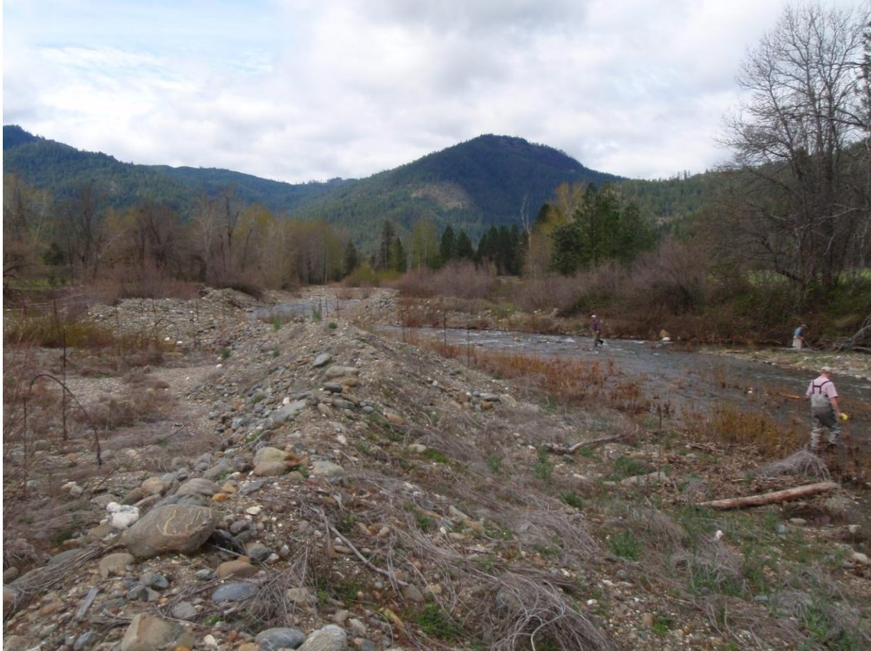
Figure 3. Flood control berms along lower Seiad Creek currently constrict the historic floodplain, blocking fish access to important rearing habitat. A collaborative project between the Karuk Tribe, MKWC and landowners would remove these berms and restore connectivity to these habitats, while protecting community resources at risk. Photo: Will Harling, MKWC.
