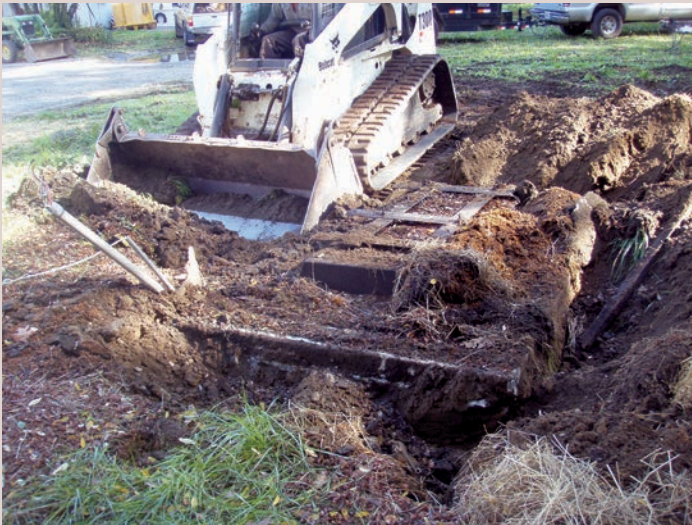
Breaking Ground at contaminated site.
