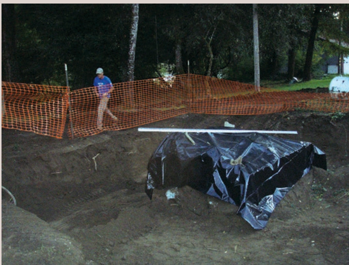
Michael Stearns fencing off dug out site.
