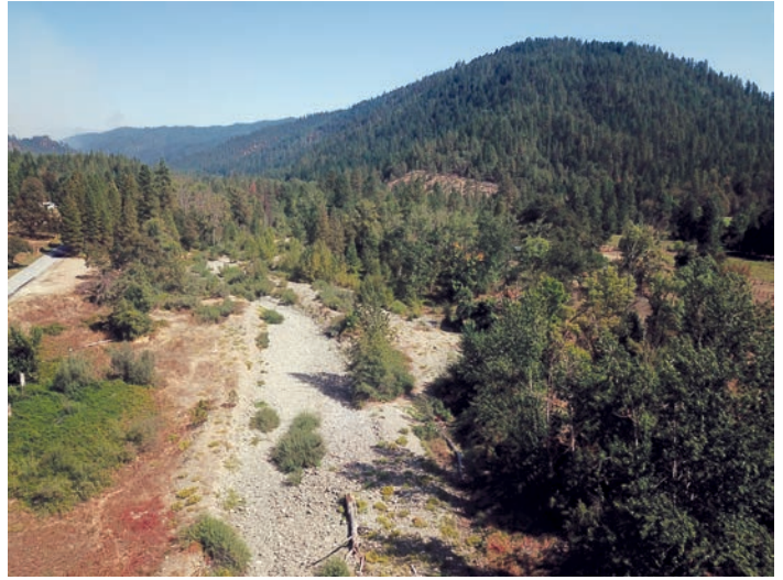
Seiad Creek Floodplain before restoration photo by Charles Wickman
