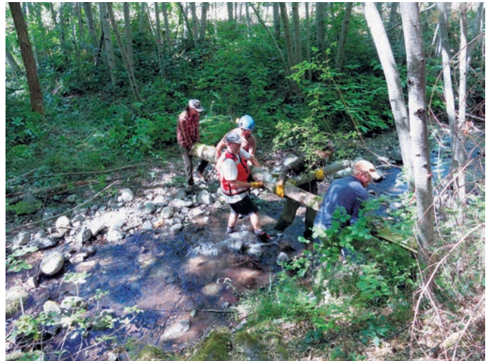
Crew anchoring a log between alder trees. photos this article by Jimmy Peterson
