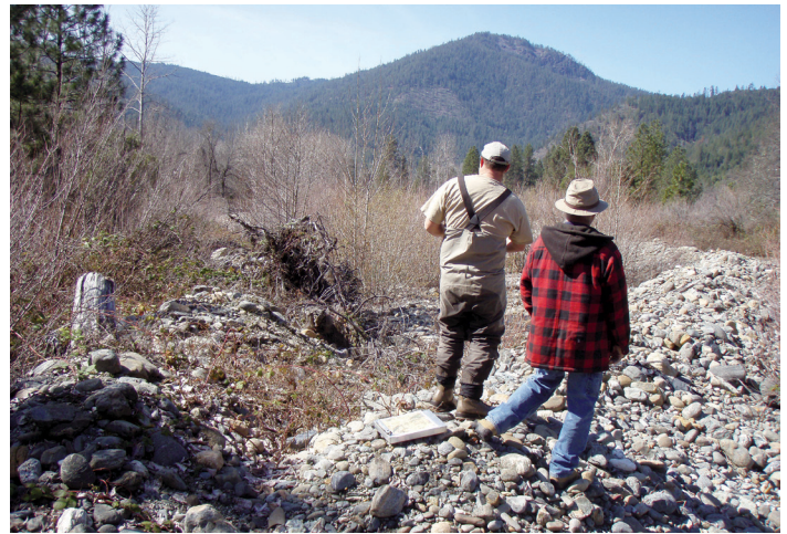
Karuk Fisheries Biologist Toz Soto and landowner Al Durazo examine the levee constructed in 2006 (right) after the Durazo residence nearly flooded, as well as past levees constructed in 1997 (left) and 1964 (farther left, not shown).
