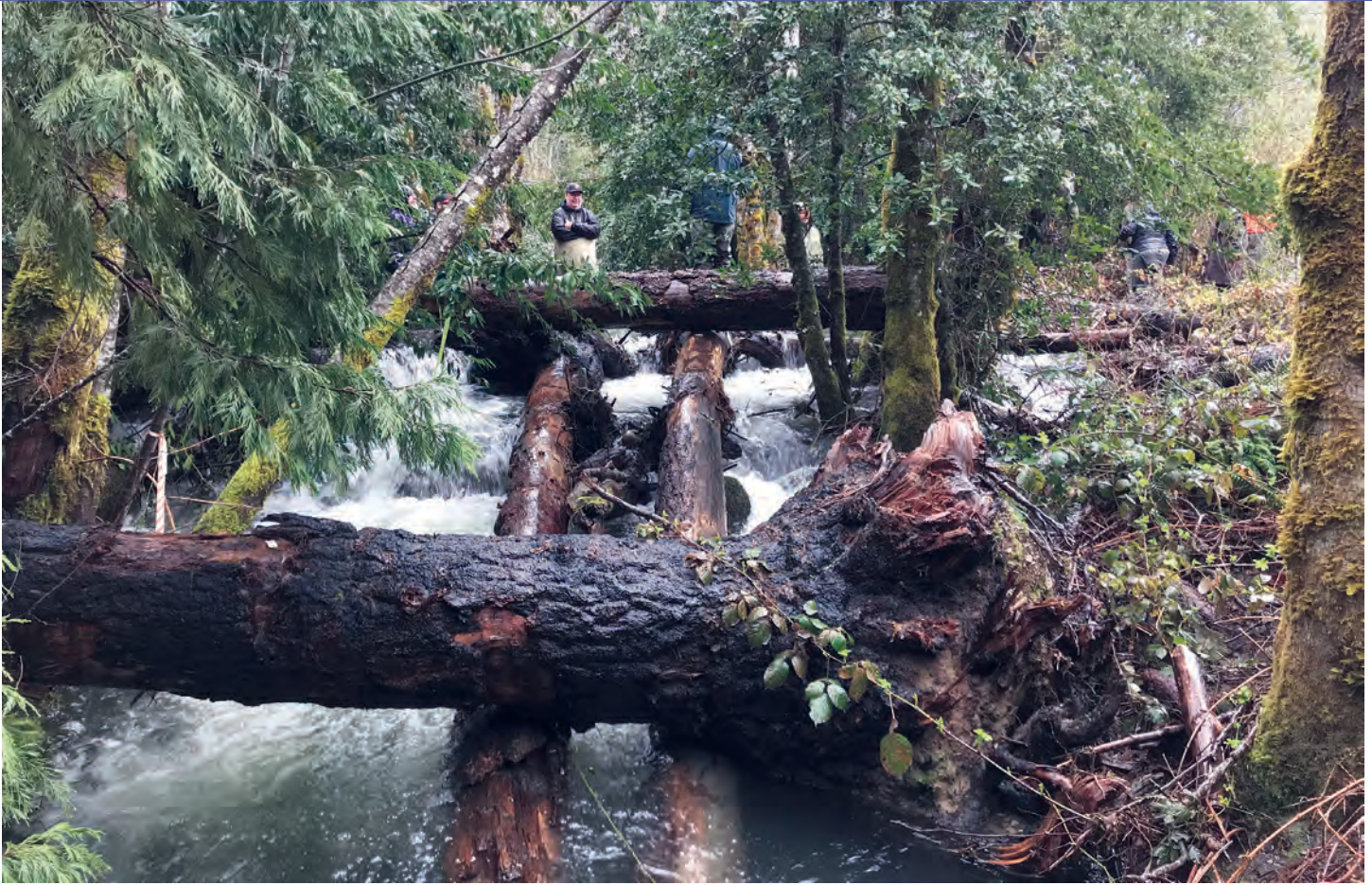
April 7, 2023. Aikens Creek Wood Structure #21 site, this photo was taken from downstream of the structure, looking upstream. This photo shows how the creek flows around the wood structure, creating multiple fish passage routes. Leroy Cyr (Six Rivers National Forest Service) can be seen in the photograph.
