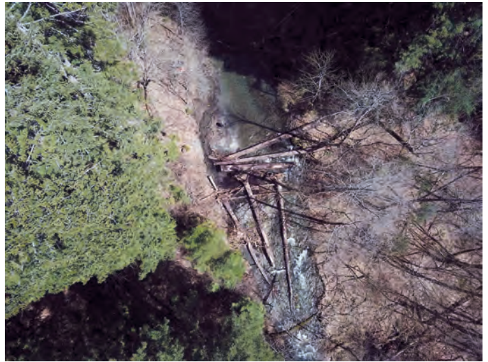
April 14, 2023. Horse Creek Wood Structure #5, from the air, in the project reach upstream of Salt Gulch, showing how the wood structure creates pockets of slow moving water for small juvenile fish to find refuge in, when the stream is flowing high. This wood structure was added to Horse Creek in the fall of 2020. Photo by Michael Hentz.
