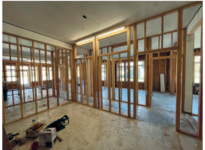
MKWC Office remodel in progress. By Carol Earnest
