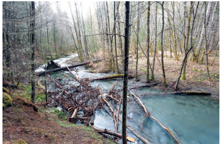
April 18, 2023. Horse Creek Wood Structure #13 site, AFTER wood structure was installed.
