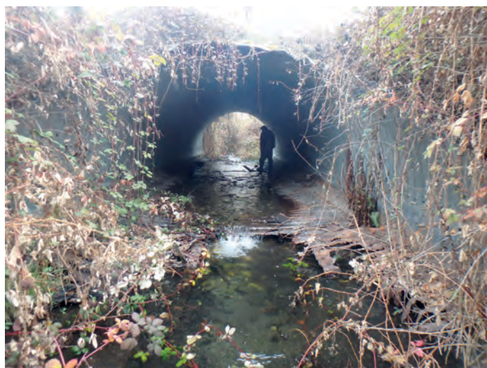
This Middle Creek culvert under Barr Road acts as a complete barrier for juvenile fish and a partial barrier for returning adult Coho Salmon. It also poses a structural threat to Barr Road.
