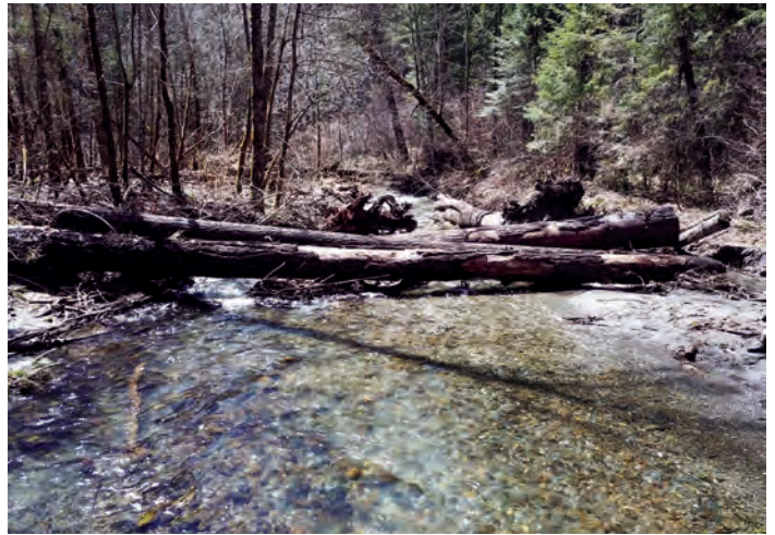
April 14, 2023. Horse Creek Wood Structure #5, on the ground, showing how the wood structure retains gravel.
