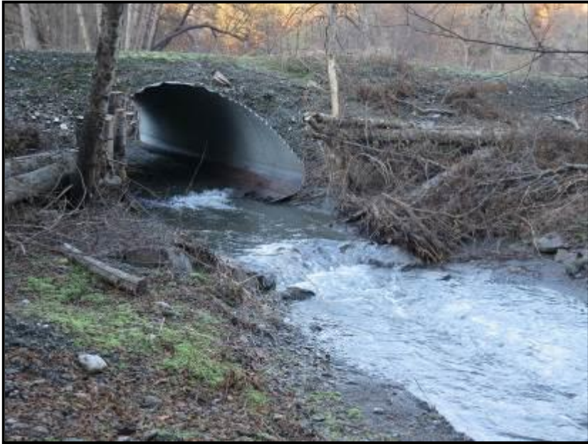
Photo 9: Culvert crossing on Middle Creek during high water event in December 2016
