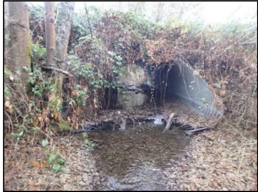
Photo 10: Culvert during low flows in December of 2015
