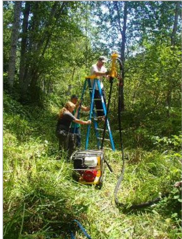
Image 1: MKWC Fisheries Staff installing ground water wells. Wells were used to monitor ground water levels throughout the year prior to construction.
