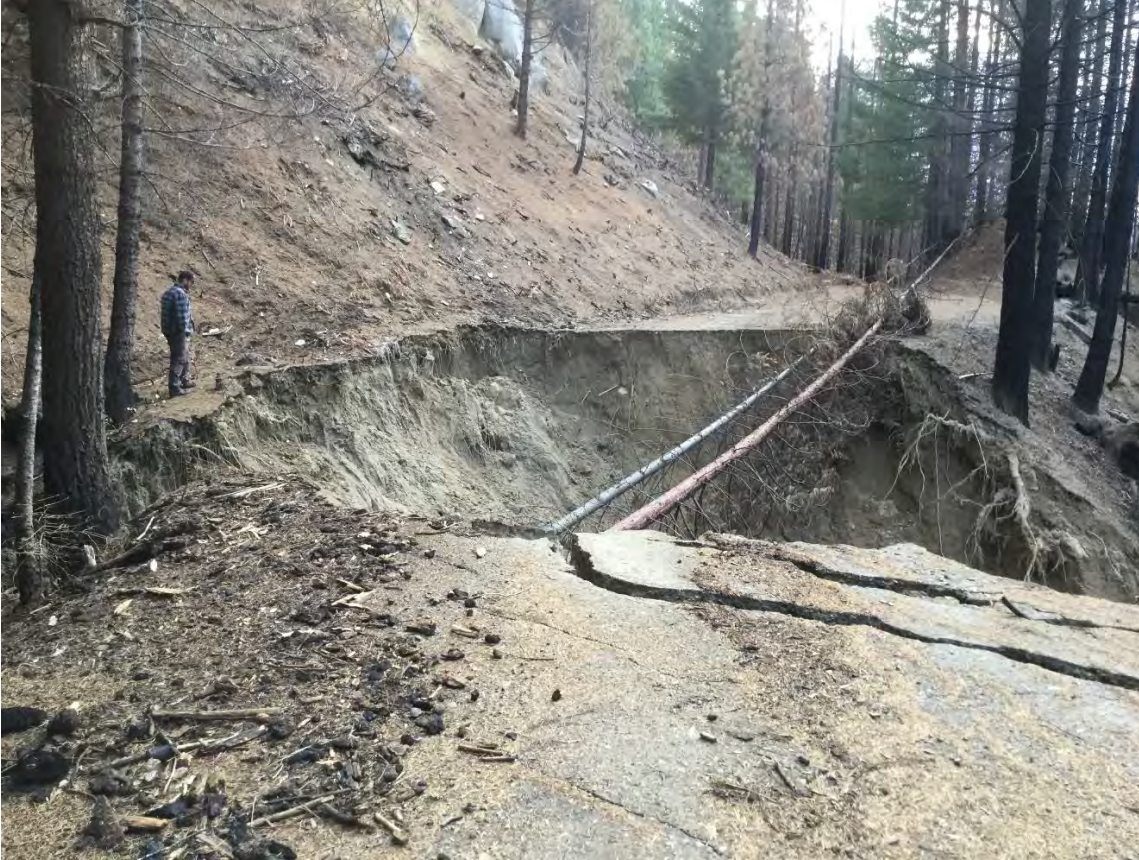
Figure 2. 15N17 failure viewed from left side (if facing downhill).
