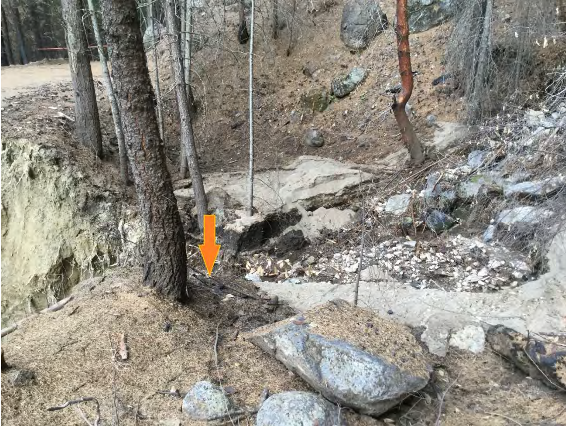
Figure 10. Right side (if looking downslope) of 15N17 road surface showing rafted debris from overtopped, water filled Inlet basin.
