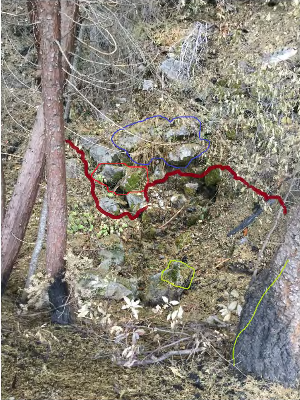
Figure 11. Left is looking upstream at boulder head of inlet basin before debris flow (Sept. 2017 during fire activity). Photos on the right were taken after the debris flow. Colors match analogous landmarks, and the dark red line shows level of sediment deposition. The inlet is about 1-2 feet downstream, and about 1.5-2 feet below the green circled boulder.
