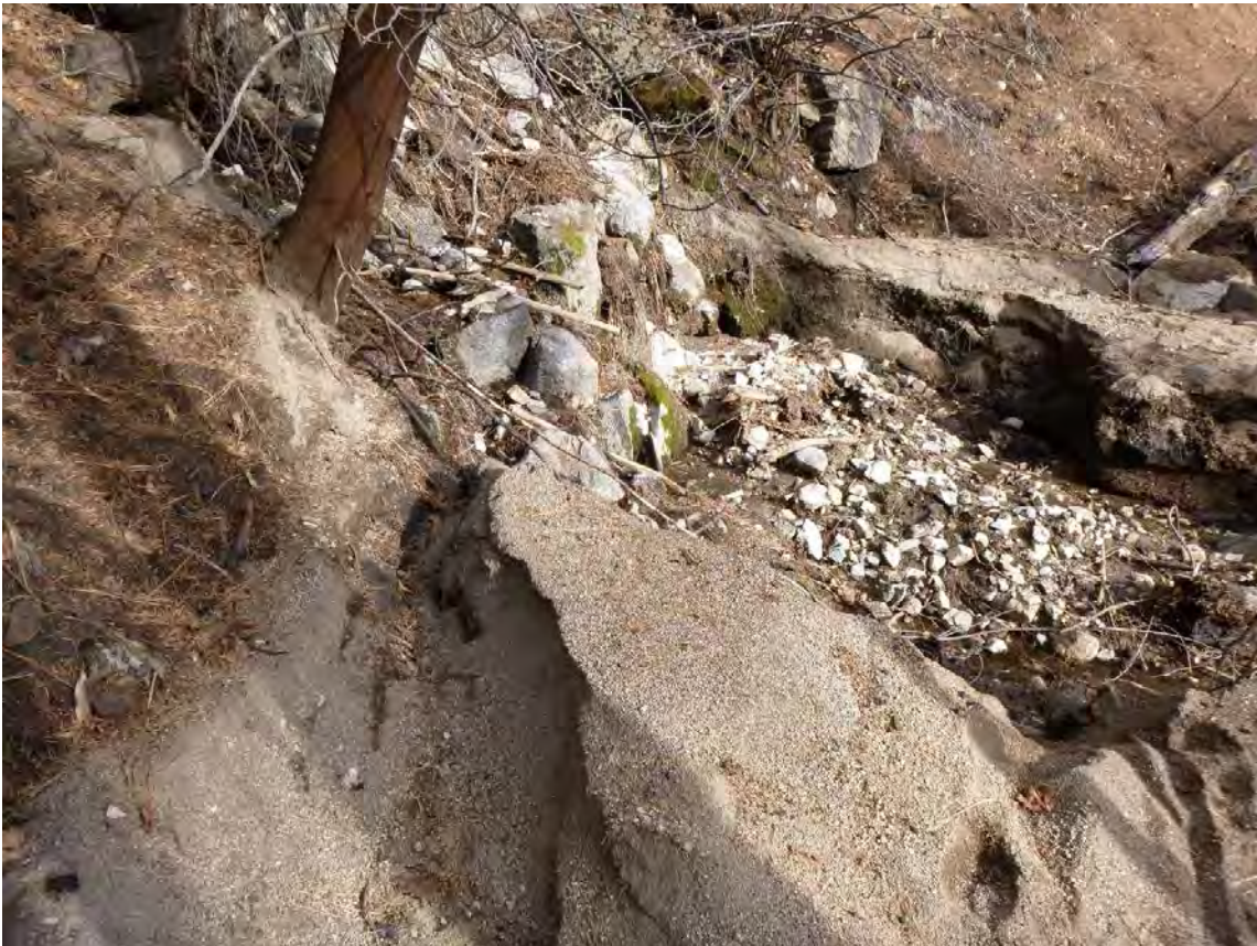
Figure 8. Close up of upstream end of 15N17 inlet basin showing 4 ft. height of sand deposition against boulder bank.
