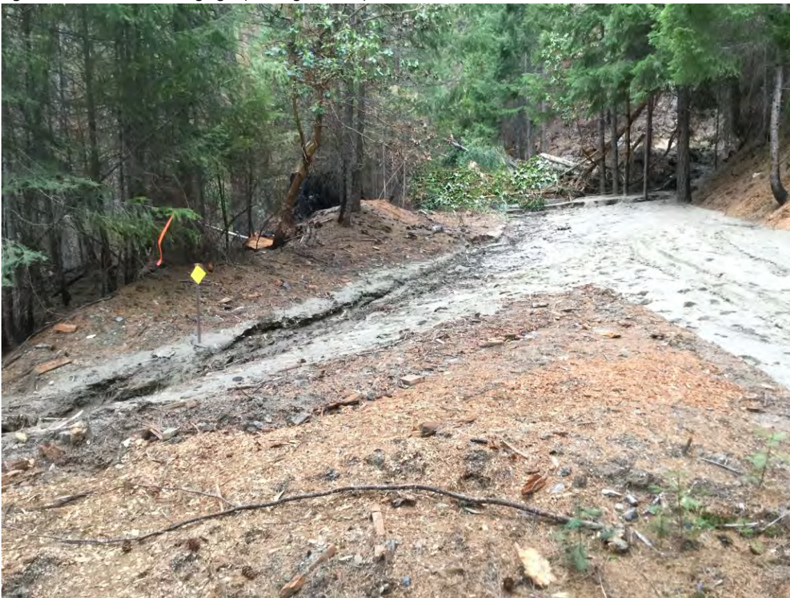
Figure 25. Closer view looking right (if facing downhill) at diverted flow and sediment from debris flow on 13N11.
