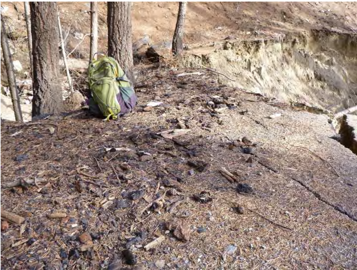
Figure 10. Right side (if looking downslope) of 15N17 road surface showing rafted debris from overtopped, water filled Inlet basin.
