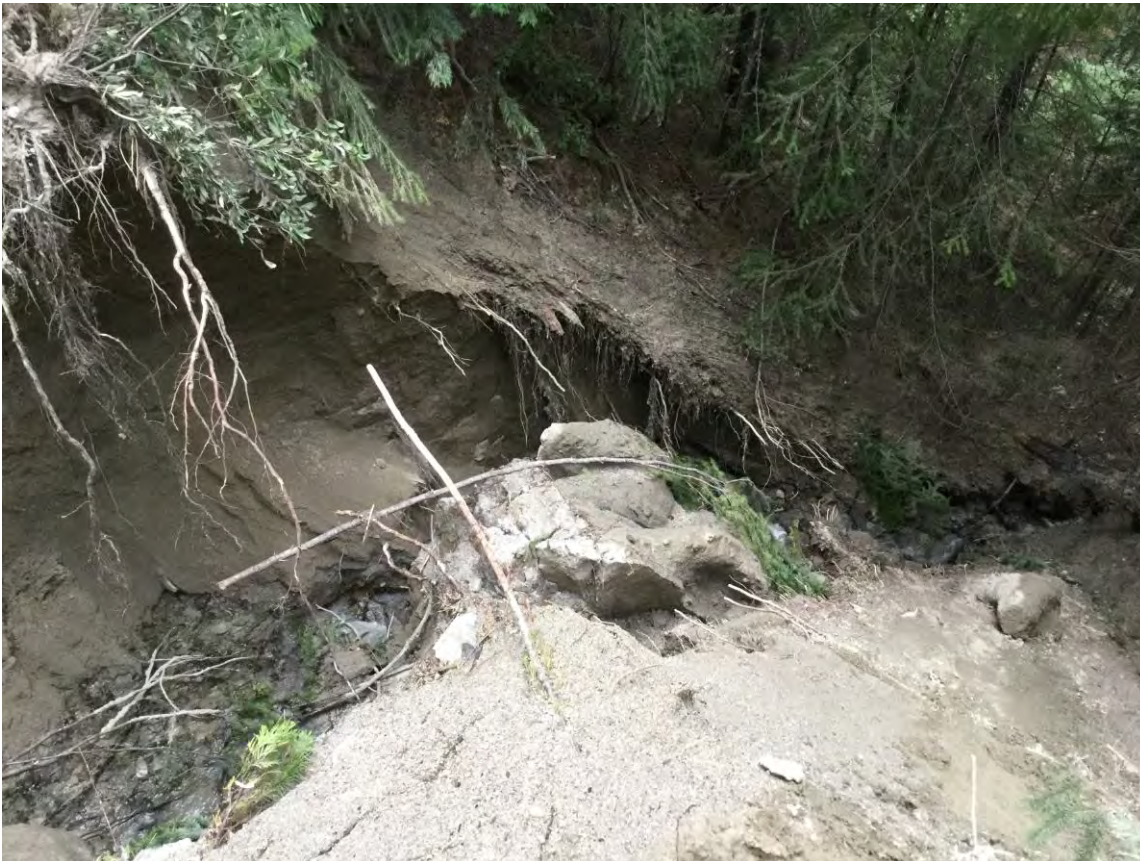
Figure 23. Looking downstream at lower end of gully and base of 13N11 fill.
