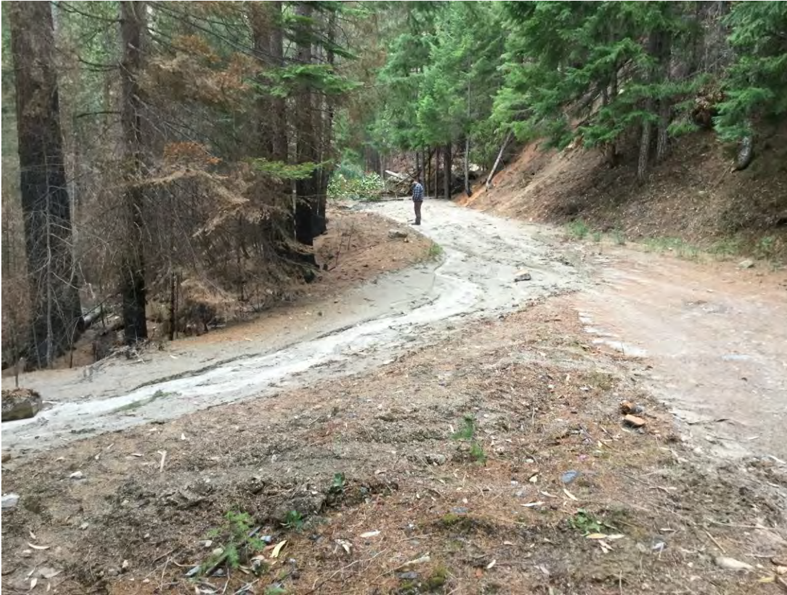
Figure 25. Closer view looking right (if facing downhill) at diverted flow and sediment from debris flow on 13N11.
