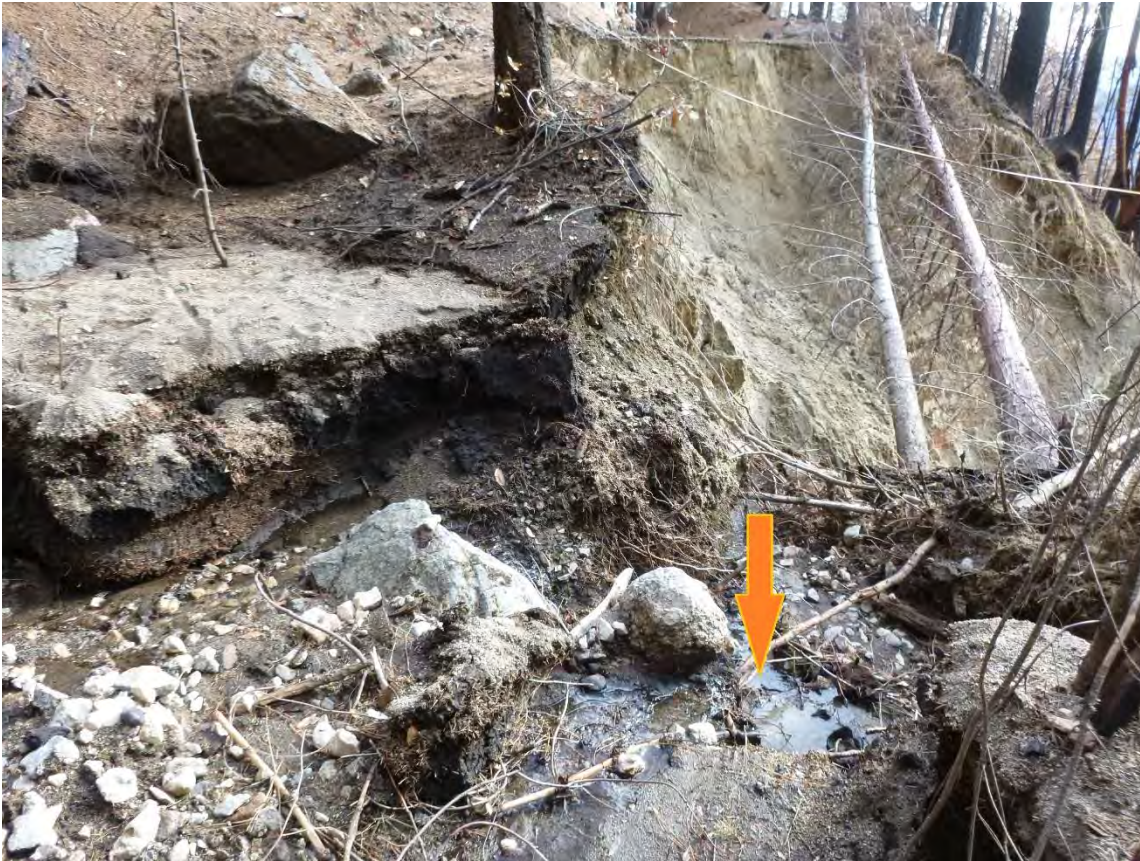
Figure 8. Close up of upstream end of 15N17 inlet basin showing 4 ft. height of sand deposition against boulder bank.
