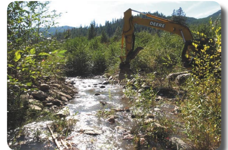
Creek Mouth Restoration at Thompson Creek
