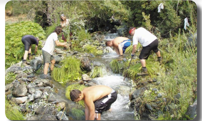
MKWC crew constructing step-pool fishways on Rogers Creek.
