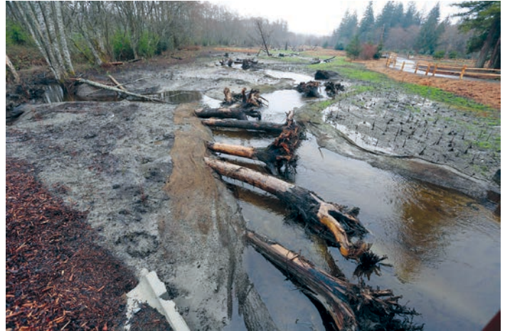
Clear Creek on the east side of the Olympic Peninsula was an example of a fish habitat restoration project that also solved a transportation issue. Every year a major street just downstream would flood due to poor water storage and drainage. By reconnecting the floodplain and establishing multiple channels, NSD has kept the road from flooding for the past three years. MKWC is currently working on several floodplain projects. photo by Will Harling
