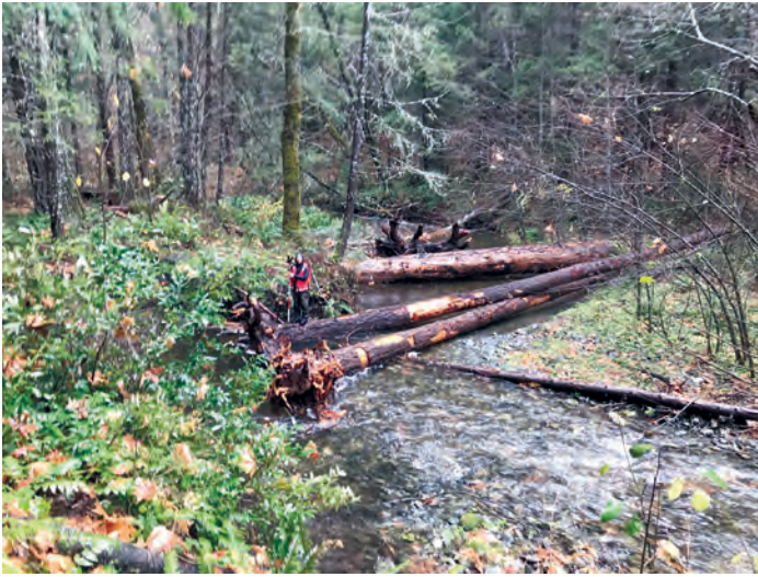
MKWC Senior Field Technician Florance Condos stands atop a completed structure.
