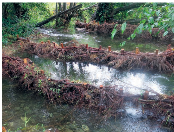
The finished BDA on Boise Creek.
