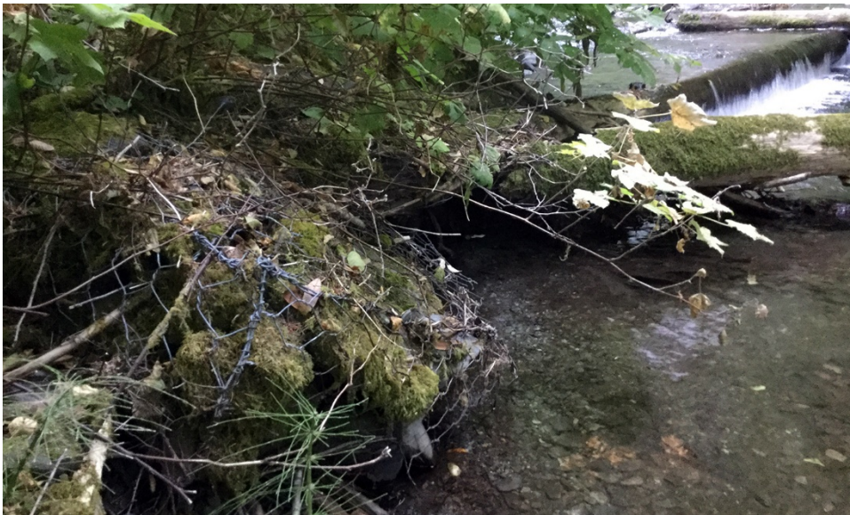
Figure 2-3. Previous restoration work completed on Cedar Creek, Lower Trinity RD. Gabion basket (cyclone-fencing baskets filled with rocks) in forefront with rebar-pinned full spanning large wood structures in background. Photo courtesy of Ely Boone.
