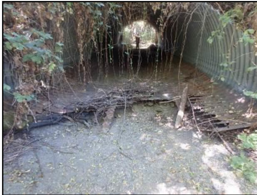
Photo 8: Dry creek channel in July of 2015
