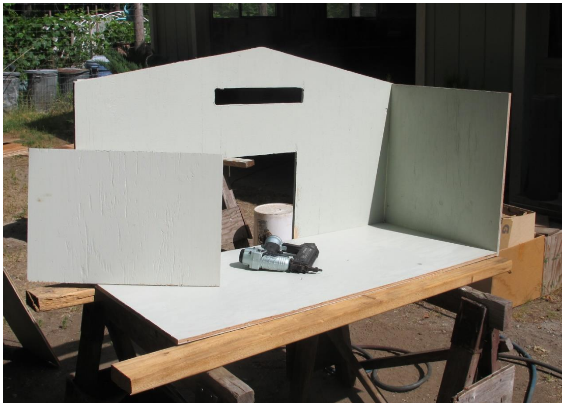
2. Join panels with small nails or brads, and wood glue.
