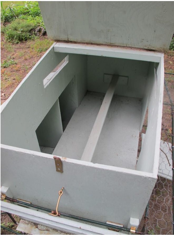
3. Add a perch inside the main room in the center along the long dimension. Note that the nesting box has a middle divider to create two sections.
